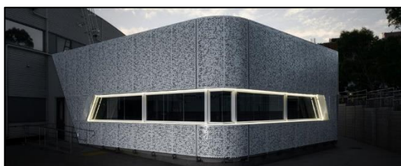
Figure 2 – ADS: Main Hall extension building for the Advanced Diffraction and Scattering (ADS) end stations. Source: ANSTO website.
